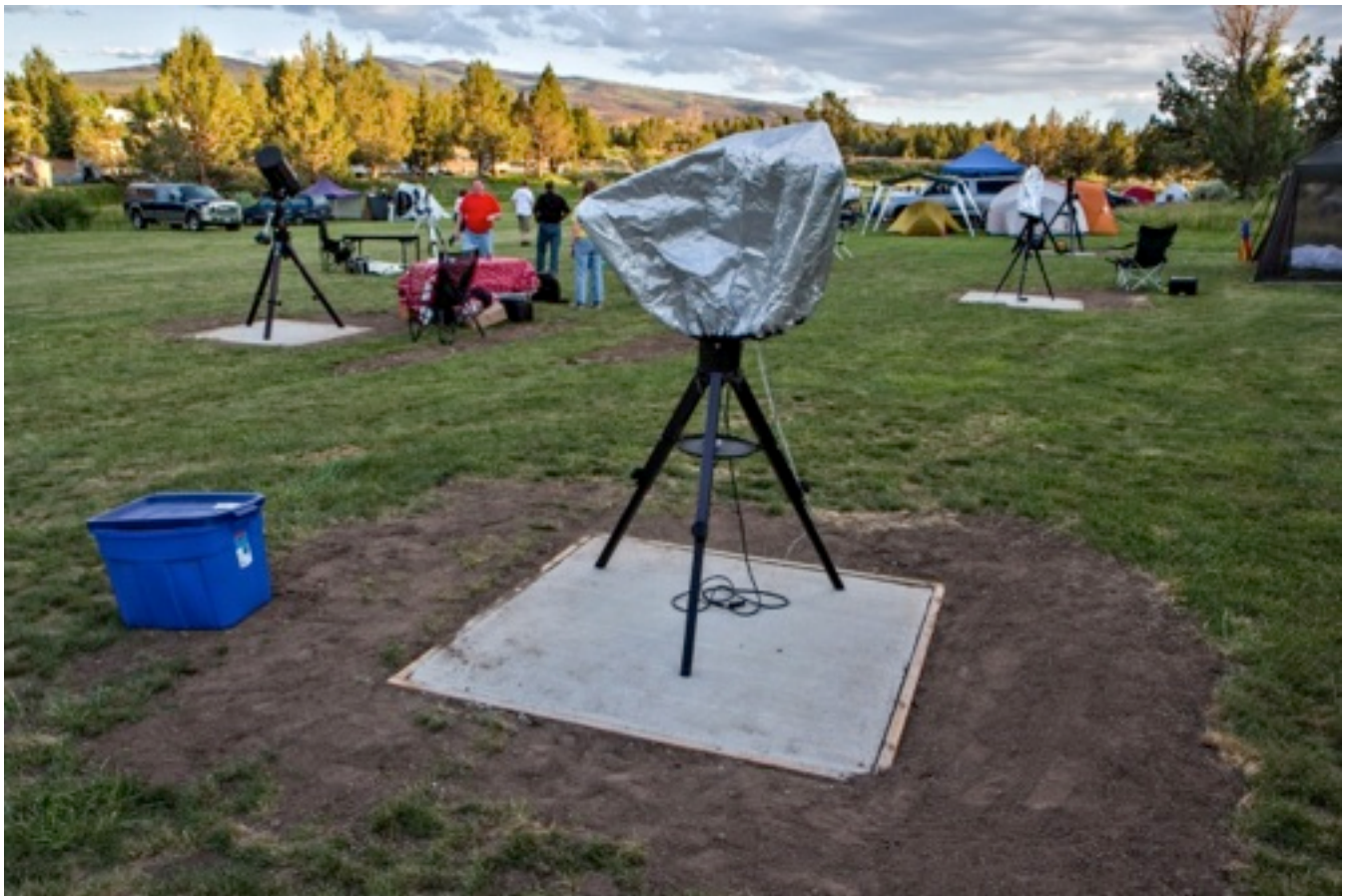
Newly installed concrete pads
